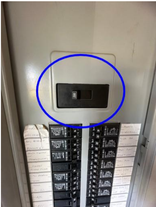
Main Electric disconnect. FYI only.
