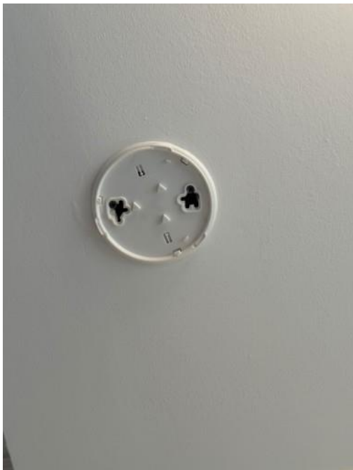
Missing smoke alarm.
