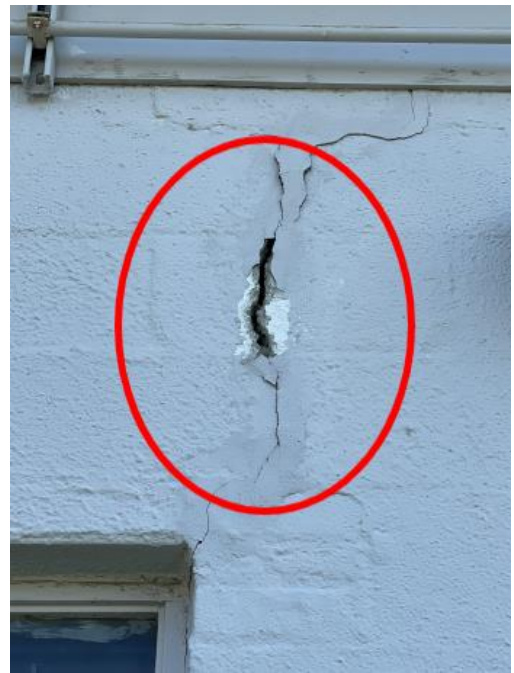
Crack and spalling Building A & B cracks Right side.
