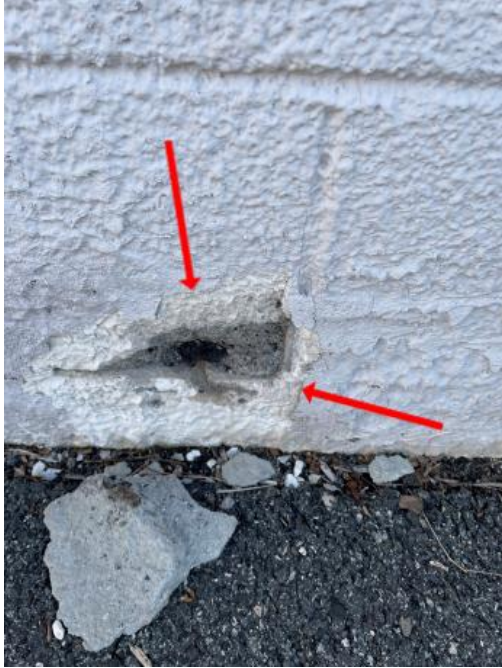
spalling Near outside condenser unit Building# C
