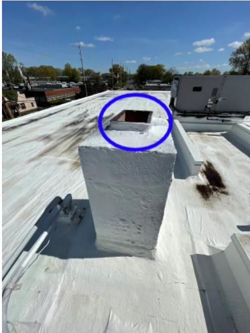
Missing Rain Cap Building A & B Roof.
