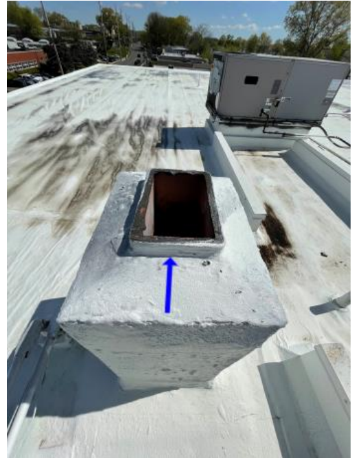
Missing Rain cap.
