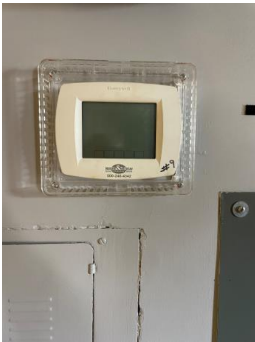
Thermostat Not responding Building A warehouse.
