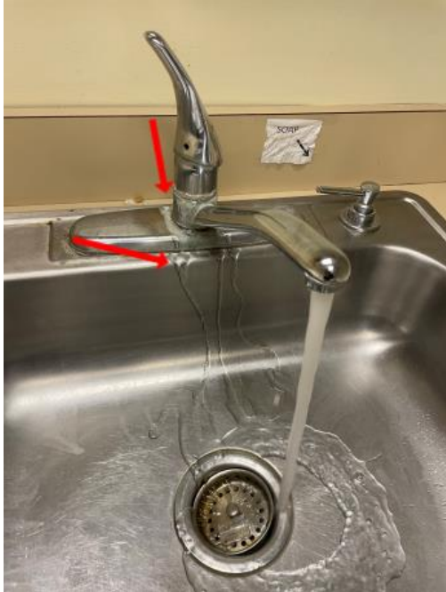
Leaking faucet upper floor kitchen.
