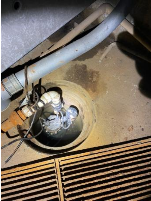
Sump Pump Building A.
