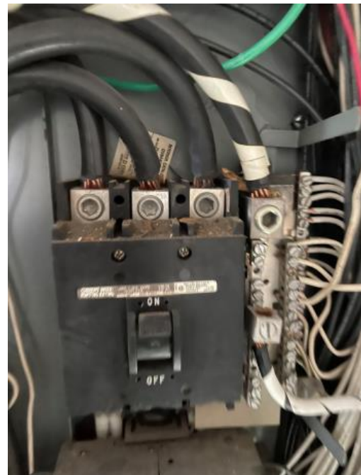
Copper main Copper branch circuits.
