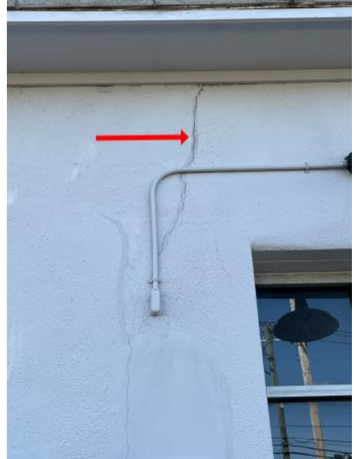
Building A & B cracks Front door.
