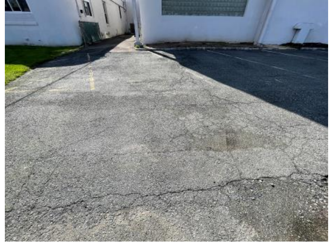
Multiple cracks on Driveway.
