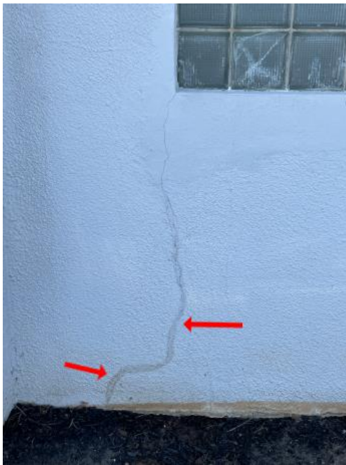
Building A & B cracks front left side.
