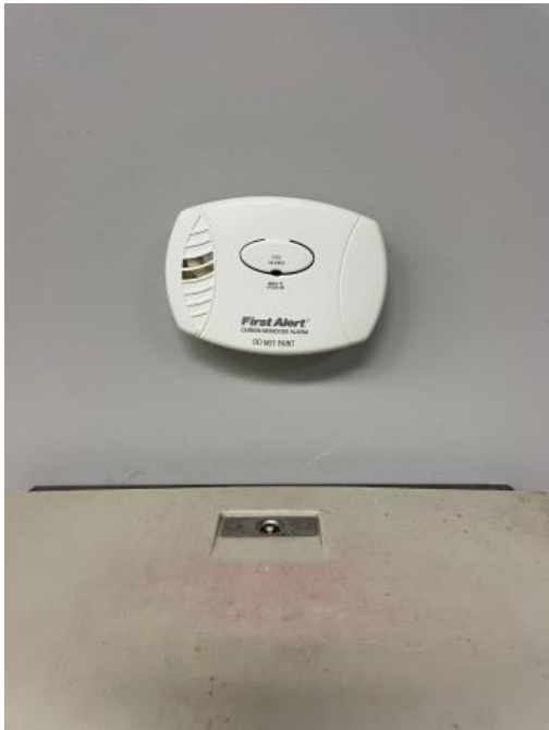
Carbon Monoxide detector.
