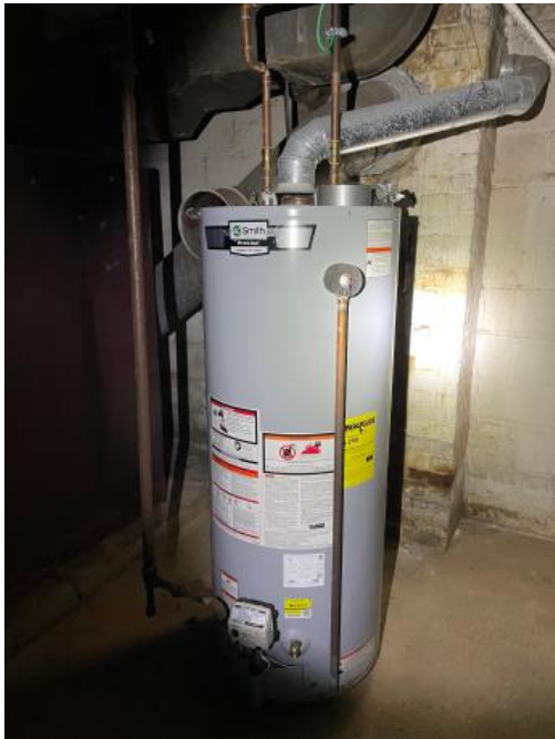
Water heater Building A .
