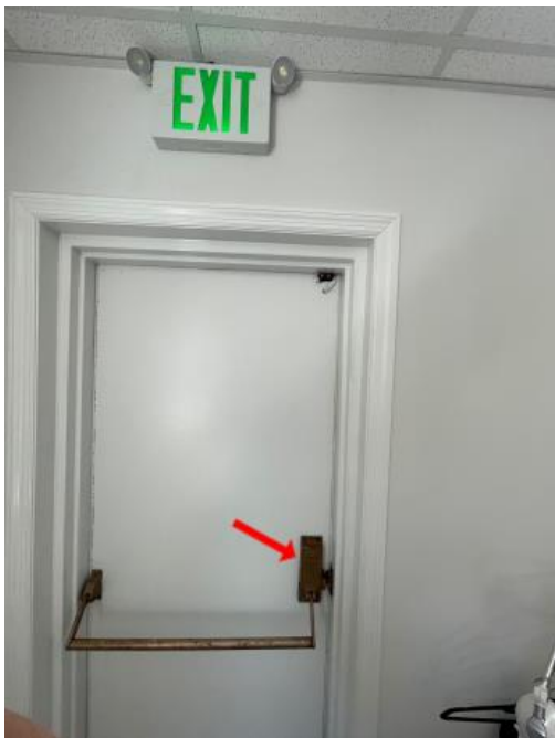
Egress lock upper floor Building C.
