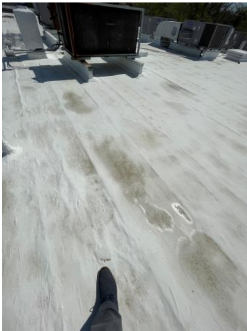
Low slope water ponding.
