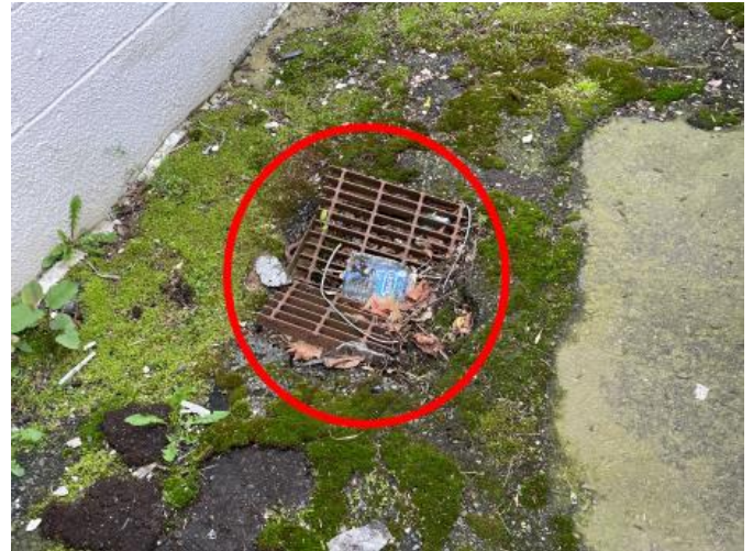
Broken or clogged Drainage.
